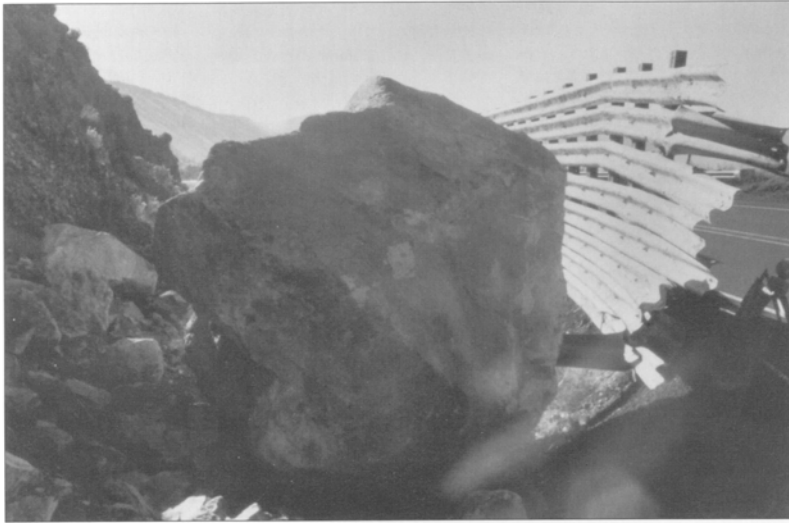
Figure 7. Close-up of large boulder from the Modoc Rim rock slide (Figure 6) that breached barrier along U.S. Highway 97.
