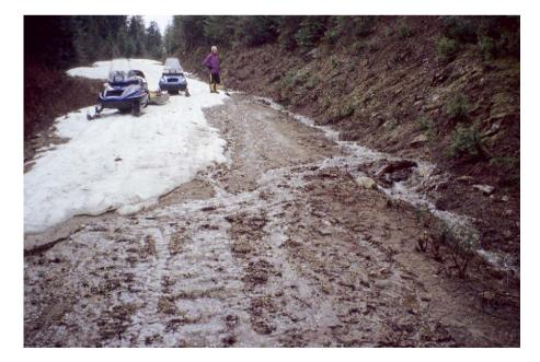
Fig. 11. Most of the development-related sediment in Redfish Creek watershed comes from erosion of the road surface and ditches during snowmelt runoff. Road surface erosion can be estimated by measuring the dimensions of eroded rills.
