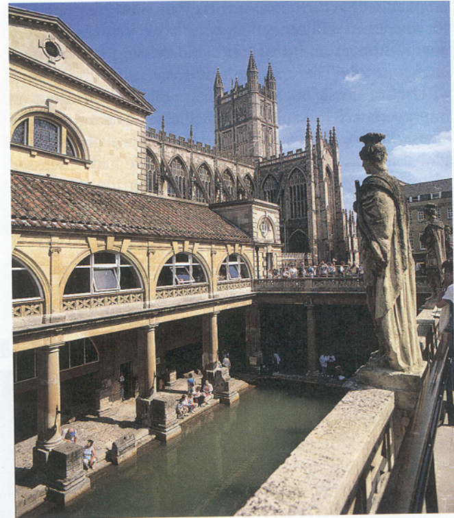
Figure 16.1 • Roman bathhouse (lower level) in the town of Bath, England. The orientation of the bathhouse and the placement of windows are designed to maximize the benefits of passive solar energy.
