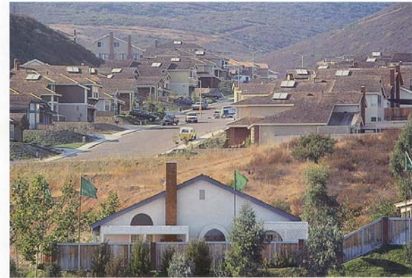
Figure 14-2 Rooftop hot water. In warm climates, solar hot-water heaters are becoming commonplace. Note the solar water-heating panels on each of the homes in this development in southern California.
