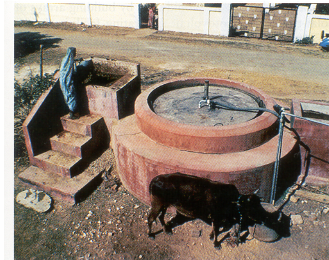
Figure 14-20 Biogas power. Animal wastes are introduced to this unit in rural India and mixed with water. The wastes then decompose under anaerobic conditions, producing biogas.
