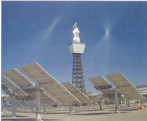
Figure 14–15 Power tower Solar Two. Sun-tracking mirrors are used to focus a broad area of sunlight onto a molten-salt receiver mounted on the tower in the center. The hot salt is stored or pumped through a steam generator that drives a conventional turbogenerator.
