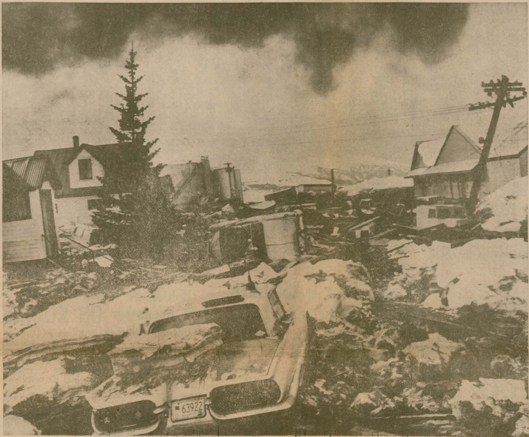
Gov. Egan's Home On Left Faces Valdez Street Of Destruction
