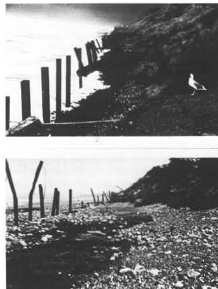
Figure 28. Progressive erosion of Cape Lookout State Park following the 1982-83 El Niño. (upper) Destruction of log bulkhead and initiation of dune erosion during October 1984. (lower) Erosion during winter of 1988, leaving a beach composed of cobbles and gravel rather than sand, and I-beams of log bulkhead at mid-beach. From Komar and others (1988).
