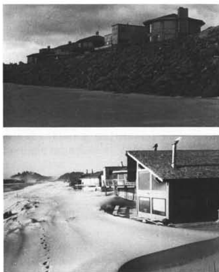
Figure 19. Upper photo: Riprap placed to protect homes under construction at Kiwanda Beach on Nestucca Spit in response to erosion during February 1978. Lower photo: Subsequent accumulation of dune sands, completely covering riprap and becoming a problem for homes (1988 photo).
