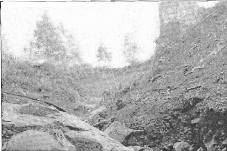
↑ Figure 7. Small initiating landslide.
