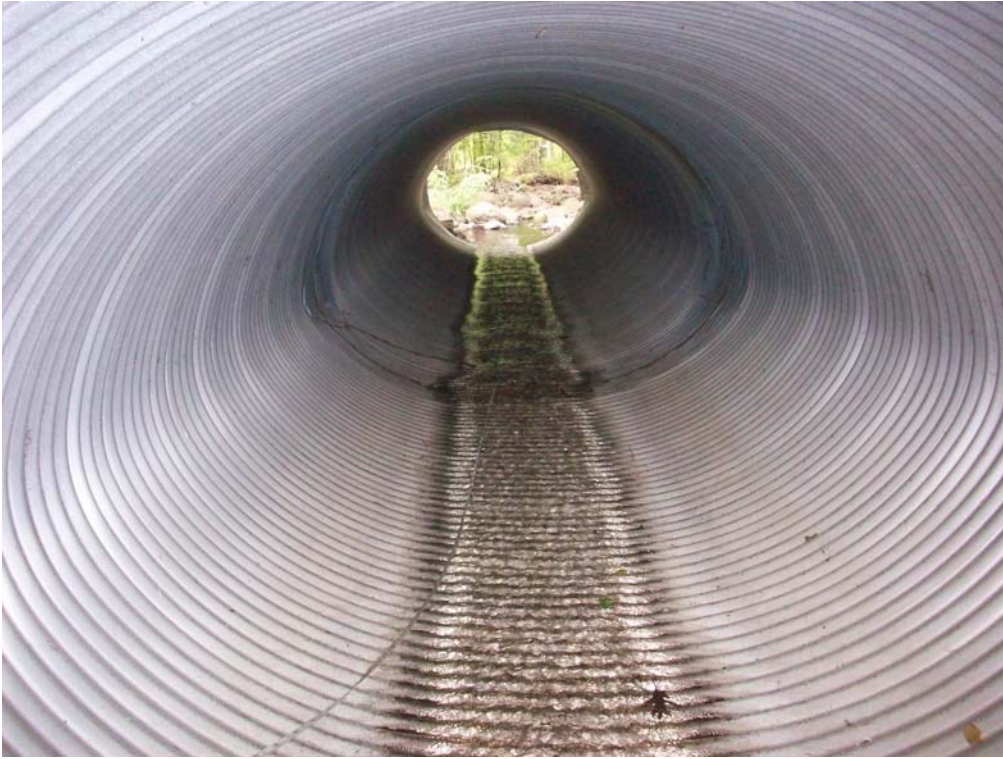
Photo 5. Site 75 predicted to be a 100% velocity barrier to juveniles; notice no objects present to retard velocity.
