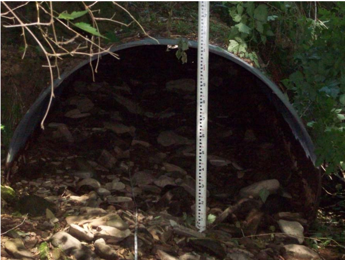
Photo 3. Site 21, stream simulated design predicted to be a 100% juvenile barrier because of velocity.
