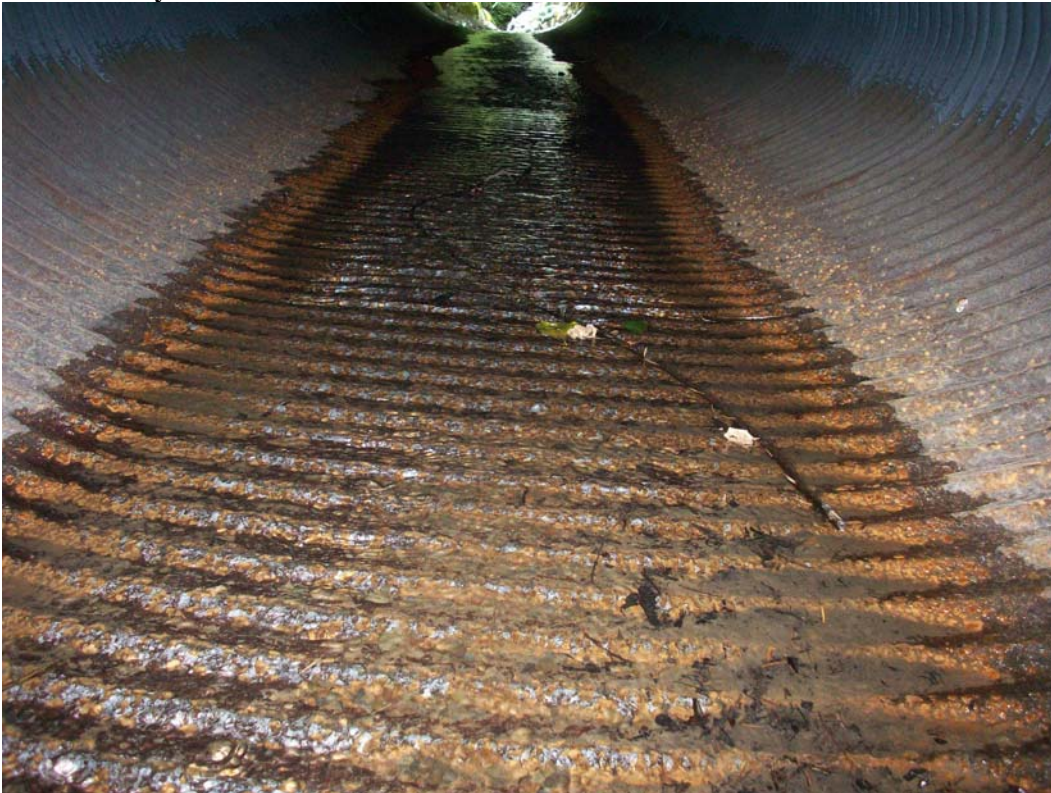
Photo 5. Site 75 predicted to be a 100% velocity barrier to juveniles; notice no objects present to retard velocity.
