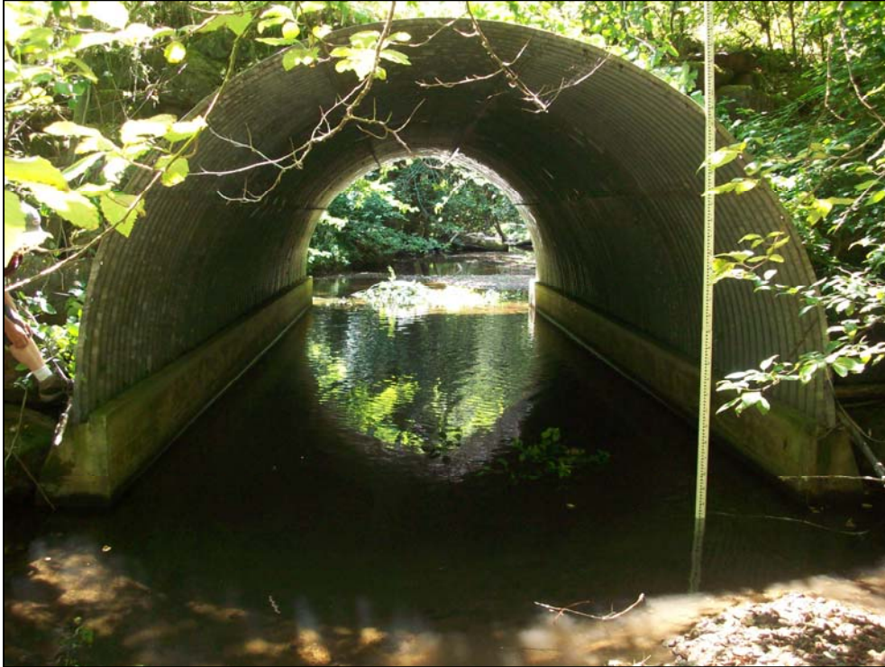
Photo 1. Site 11 bottomless arch rated as allowing juvenile to pass through only 1.8% of the modeled flows.
