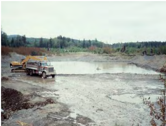
(b) Dismal Pond site during construction.
