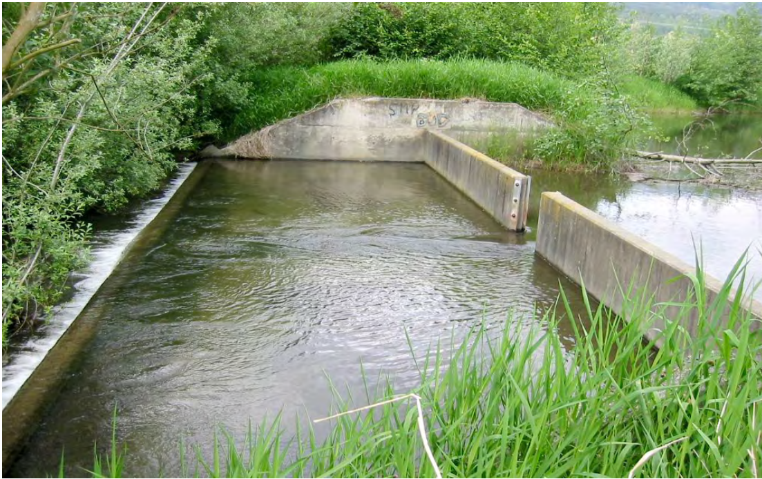
Instream Sediment Detention Basins Figure 3: Coal Creek sediment basin, detail of outlet structure. Downstream weir prevents erosion of channel. A more fish-friendly structure downstream of the slot might be a porous weir. Fish passage is an important consideration in the design of outlet structures.
