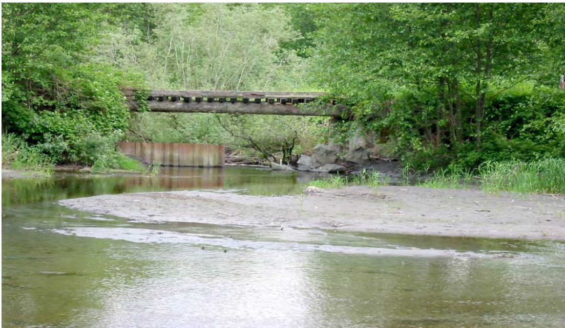
Instream Sediment Detention Basins Figure 4: Hansen Creek sediment basin, Skagit County. Looking downstream at outlet structure. Outlet is more ad hoc than other basins and can be a passage problem at some flows. Basin is actually many acres with only the outlet shown here.
