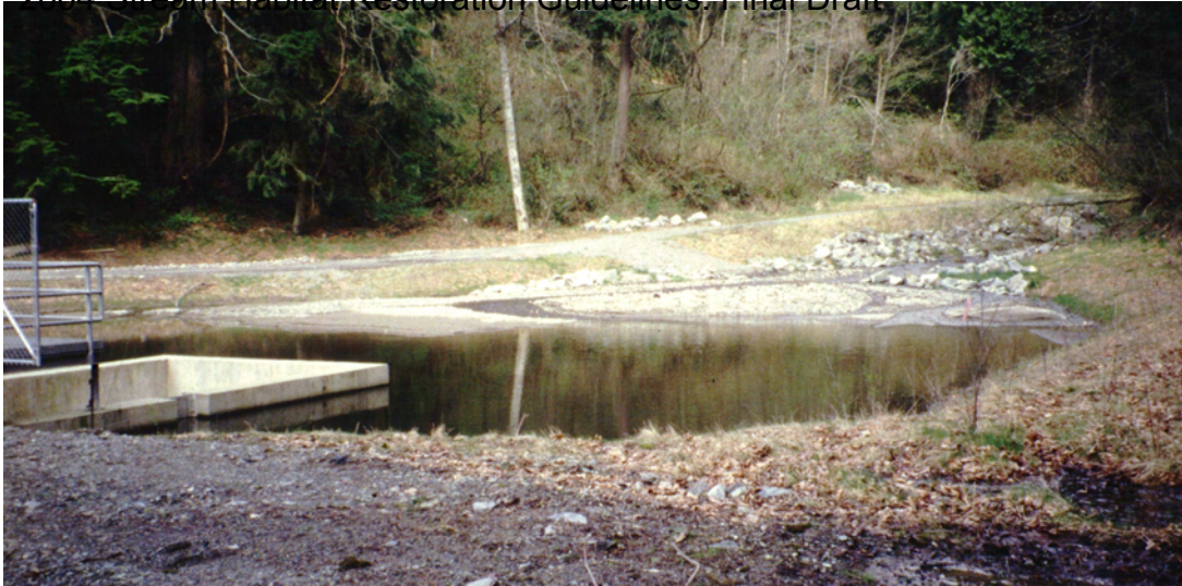
Instream Sediment Detention Basins Figure 6: Maplewood Creek sediment basin, King County. Looking upstream at sediment basin. High flow overflow structure is on right, inlet stream on right. Low flow outlet structure is a fishway off the picture on the left.
