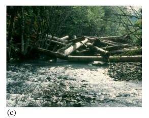
**Large Wood and Log Jams Figure 23**. Upper Finney Creek channel restoration project: (a) aerial view of placed logjams; (b) canopy closure following logjam construction; (c) logjam initiating channel re-configuration and instream habitat. (photos of Finney Creek, Skagit County, Washington, courtesy of Roger Nichols, USFS)
