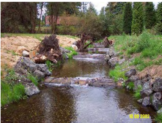
(e) Log weir grade controls. Hylebos Cr.
