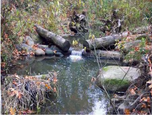
(a) K-weir. Longfellow Creek.
