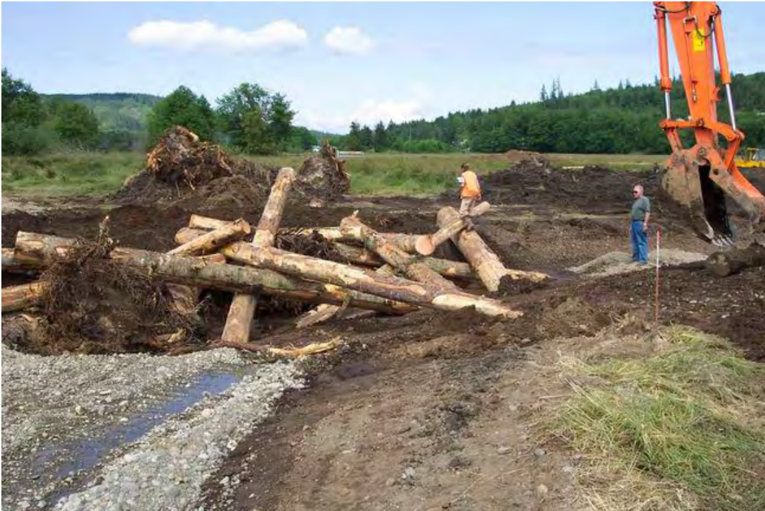
Channel Modification Figure 8: Construction of a large wood complex.
