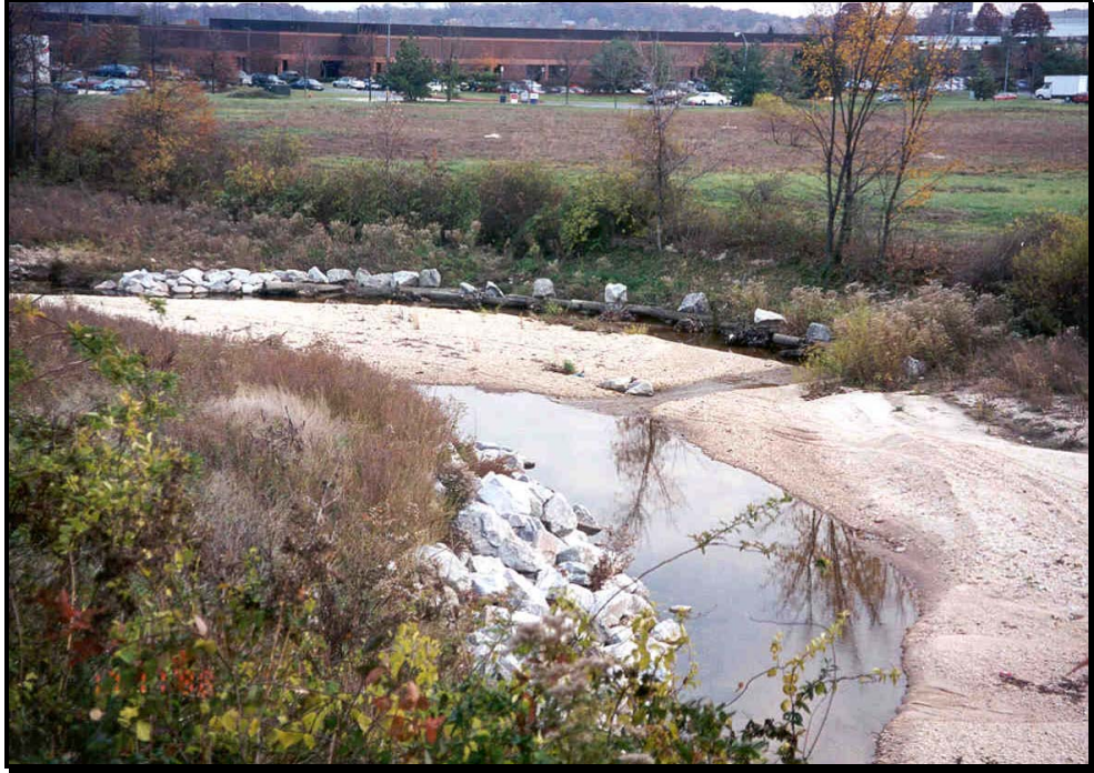
Figure 8.7 Post-project channel changes in Whitemarsh Run, Maryland, November, 1998. Sedimentation in the outer bank meander pool with outer-bank protected by rootwads in the middle of the restored reach.
