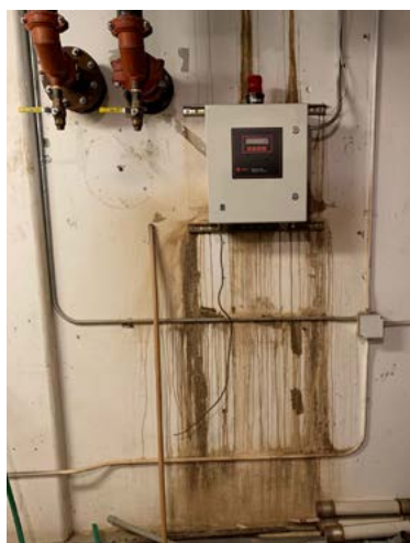
APSC deferred maintenance items: basement wall and foundation leaks, mechanical room
